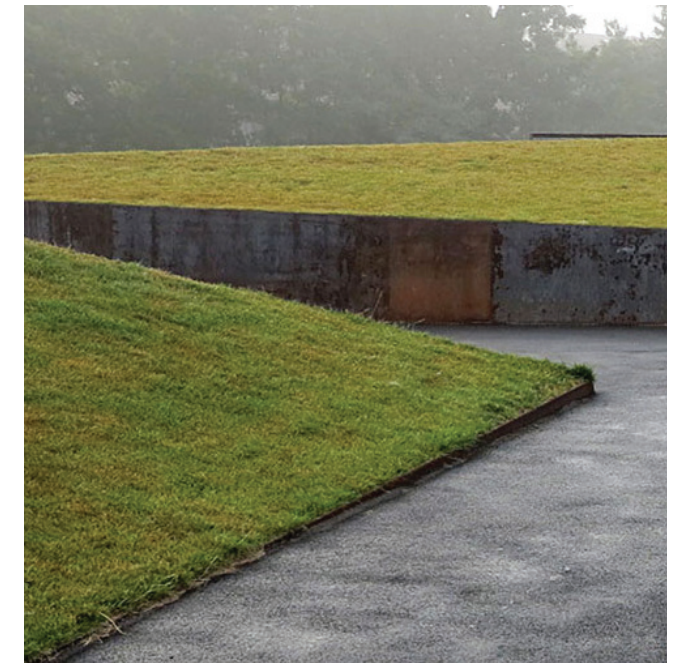
Cor-ten retaining walls at ADA Paths
