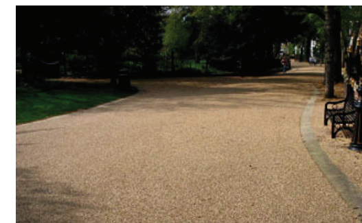
Olmsted Walk - pervious pavement with recycled concrete
