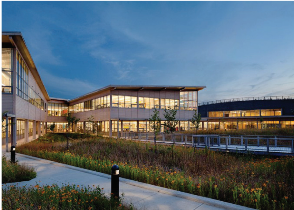
Bridge at pond edge
